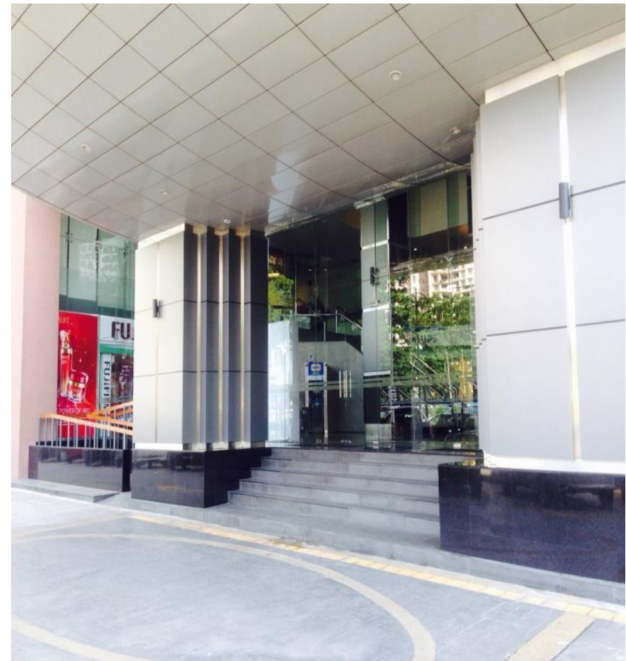
Drop-Off Area Columns
